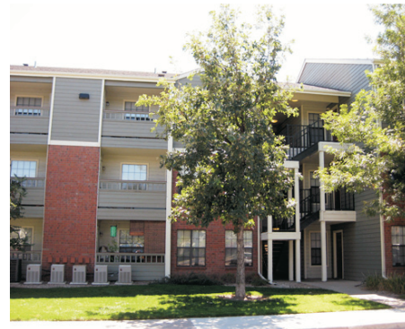
Courtney Park 4470 South Lemay Avenue (near Harmony & Lemay)
