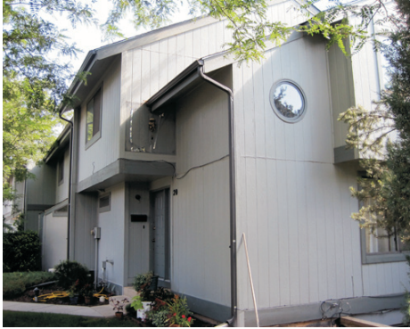
The Bridges 1610 Westbridge Drive (near Prospect & Taft Hill)
